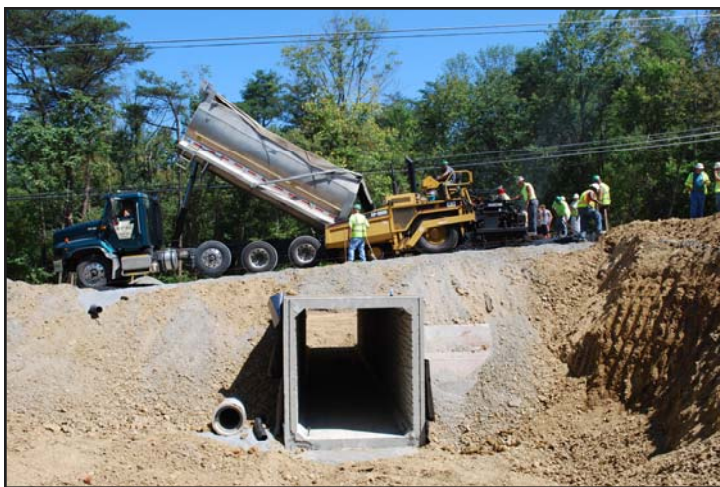
The contractor repaves PA 944 after installing the underpass. Landscaping will screen the underpass, trail, and hikers from passing motorists. Photo by Karen Lutz.
