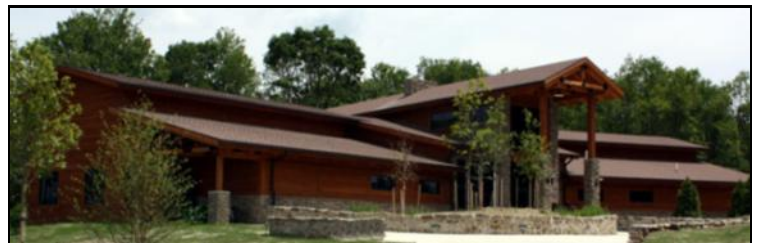
The exterior of the new Elk Country Visitor Center
