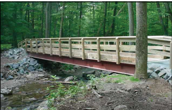
New AT bridge over Dunfield Creek in Delaware Water Gap. Photo from Ernie Kabert, Superintendent of Worthington State Forest.
