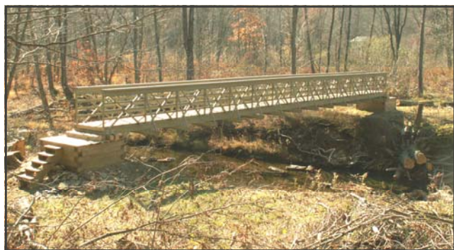
The 72 foot Corporation Dam Bridge. Photo courtesy of Ralph Seeley.
