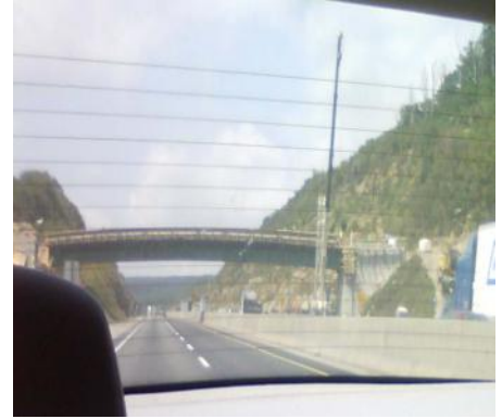
ABOVE: Laurel Highlands Hiking Trail Bridge, Courtesy of Jeff Johns, DCNR
