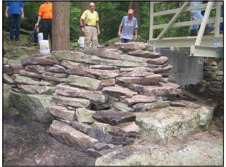
One of the rock retaining walls constructed by the August Trail Care in Promised Land State Park.
